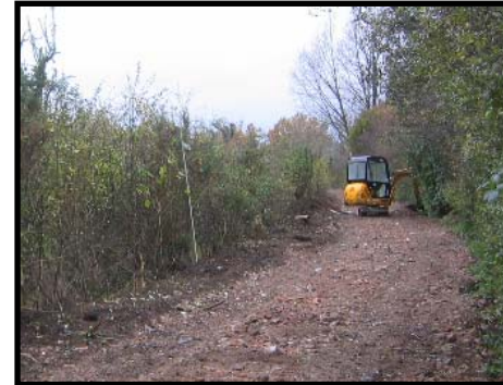
Construction of new Bridleway 25
